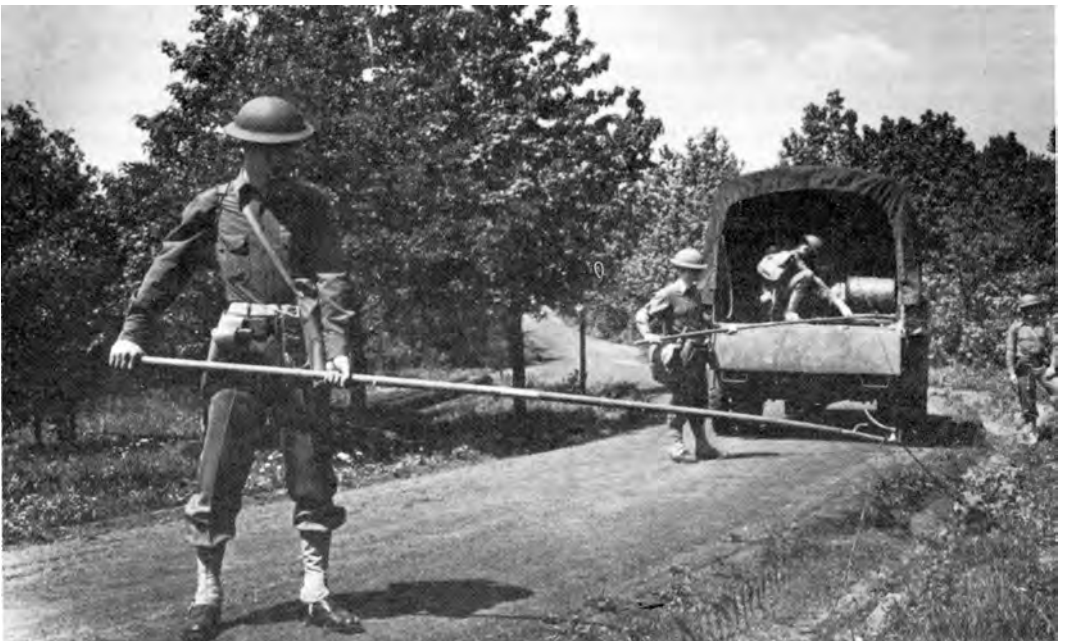
LAYING FIELD WIRE from the horse-drawn cart (above) and from the truck-mounted RL-26 (below).
