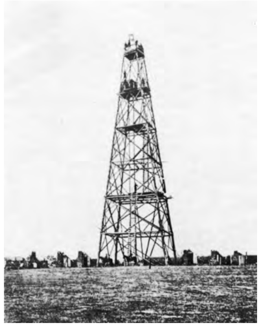
CIVIL WAR SIGNAL TOWER on Cobb's Hill, Appomattox, Virginia.
