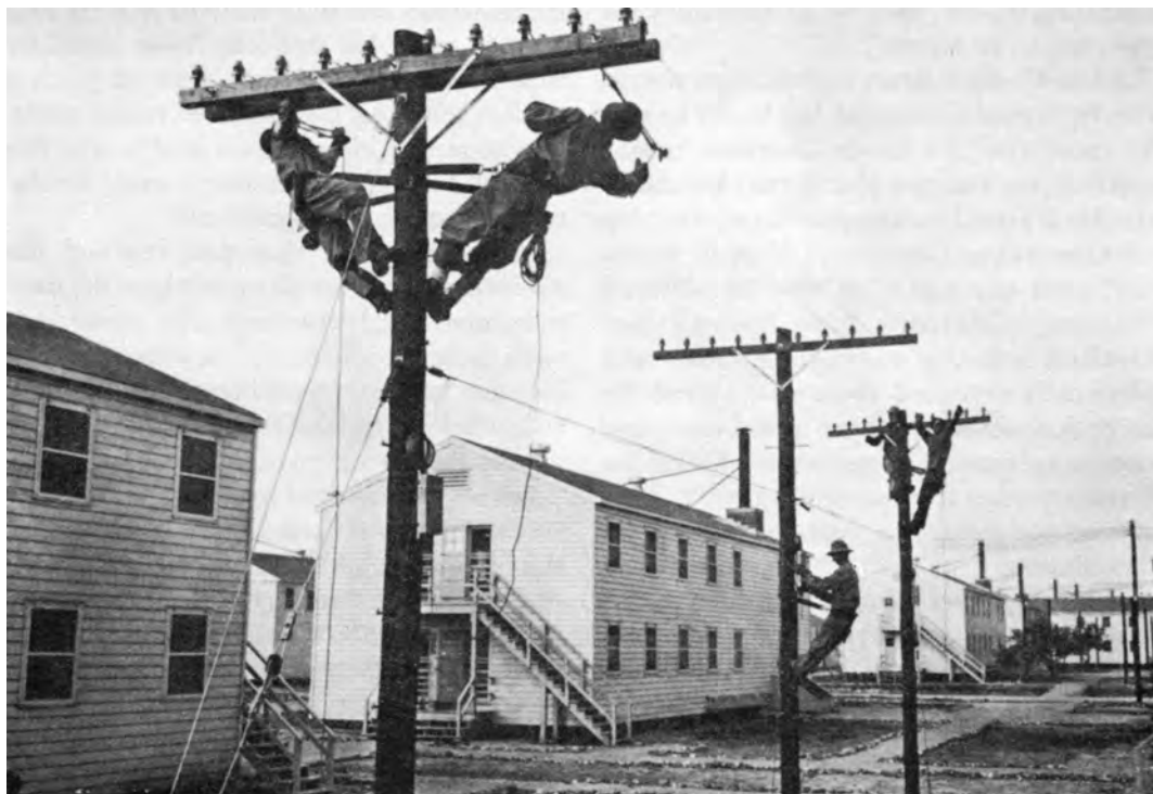
ENLISTED MEN LEARNING OPEN WIRE CONSTRUCTION. ( Photograph taken in 1942. )
