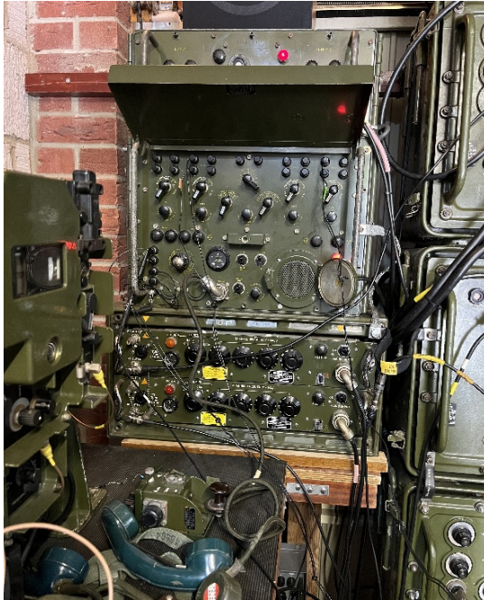
Figure 10. The carrier set telephone now installed with the C41/R222 radio relay/synthesiser equipment (although not yet connected into the terminal) and undergoing extra testing
