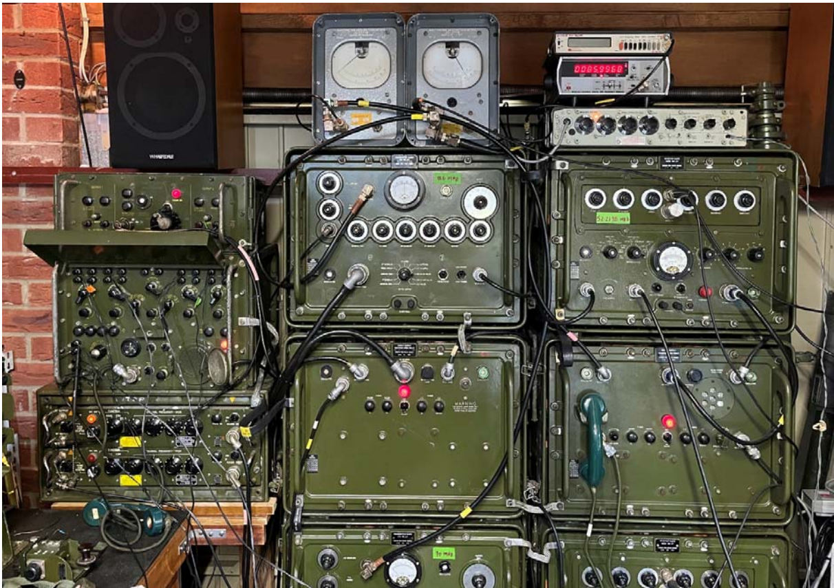
Figure 15. The final 'operational' setup of the radio relay terminal complete with frequency synthesiser and carrier set telephone/PSU
